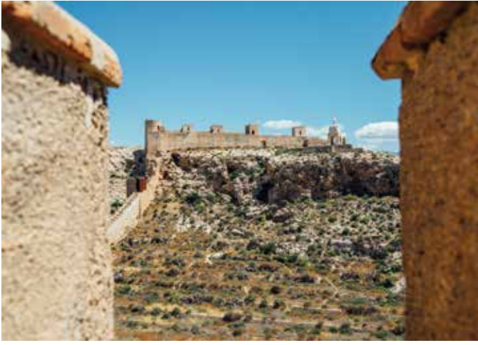
) Jayrán wall and San Cristóbal hill
